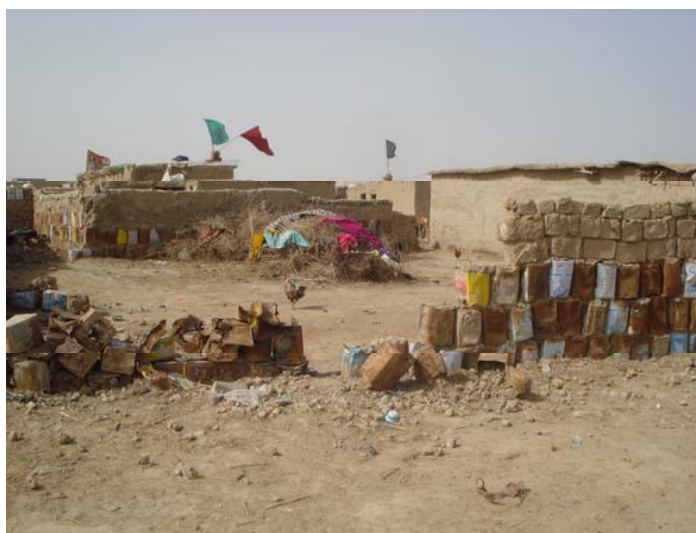
Despite improved security conditions, many IDPs are still living in substandard housing, such as in this photo, in Hay al Shuhadaa, Suwerah district, Wassit.
