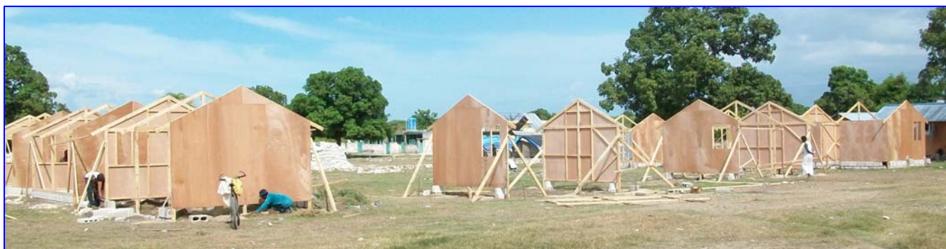
T-shelters under construction at the Defilet Buedet Psychiatric Hospital
