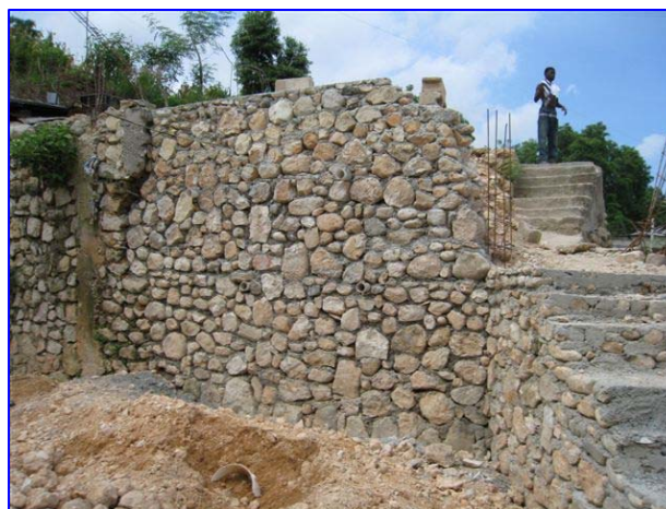
Construction of a retaining wall, Port-au-Prince, July 2010.
