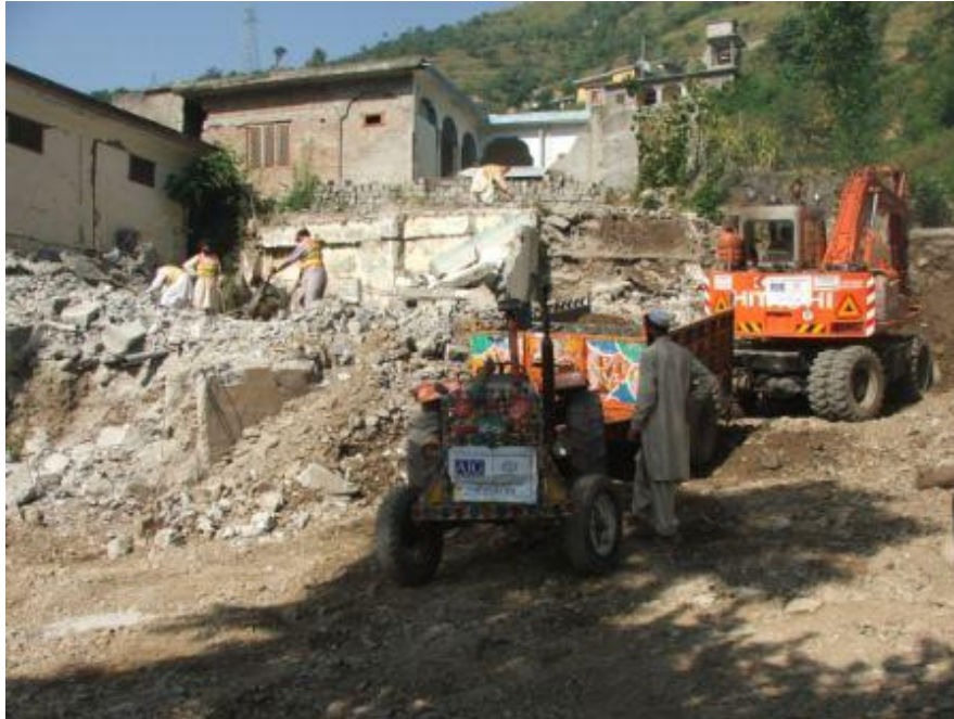
Fig 1.1 Work in progress at Chela Bandi slide
