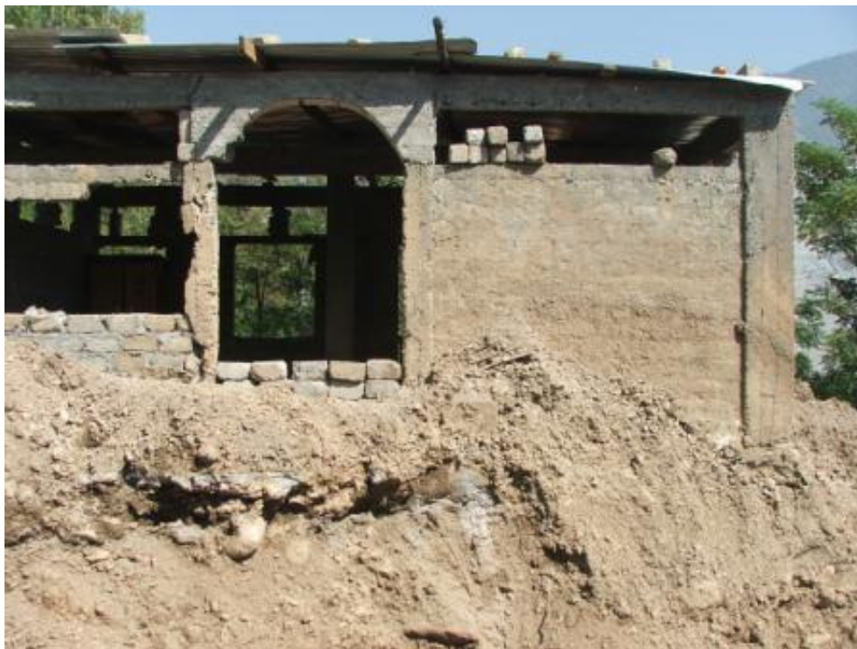
Fig 1.4 Chela Bandi Mosque after clearing
