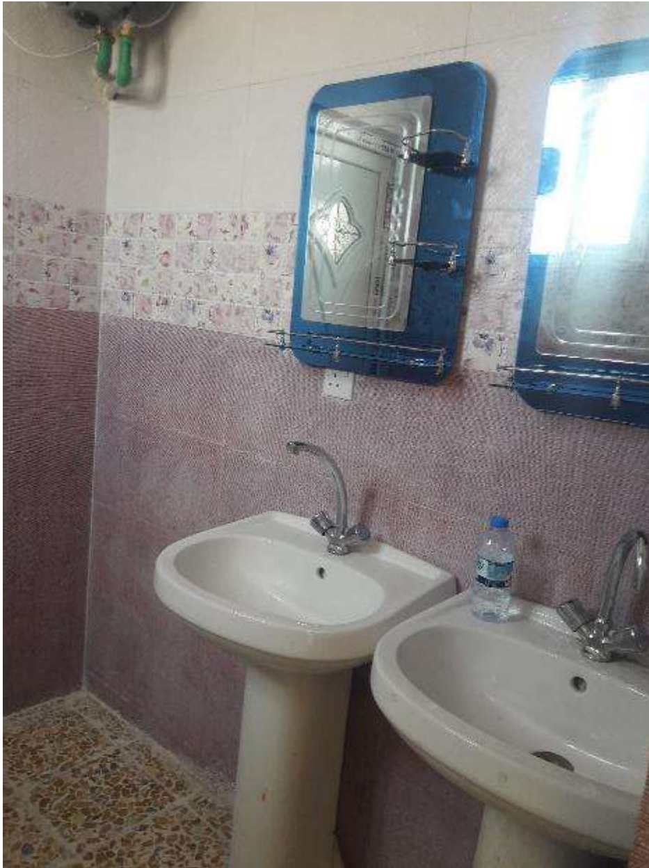
Bathroom for women in CP building
