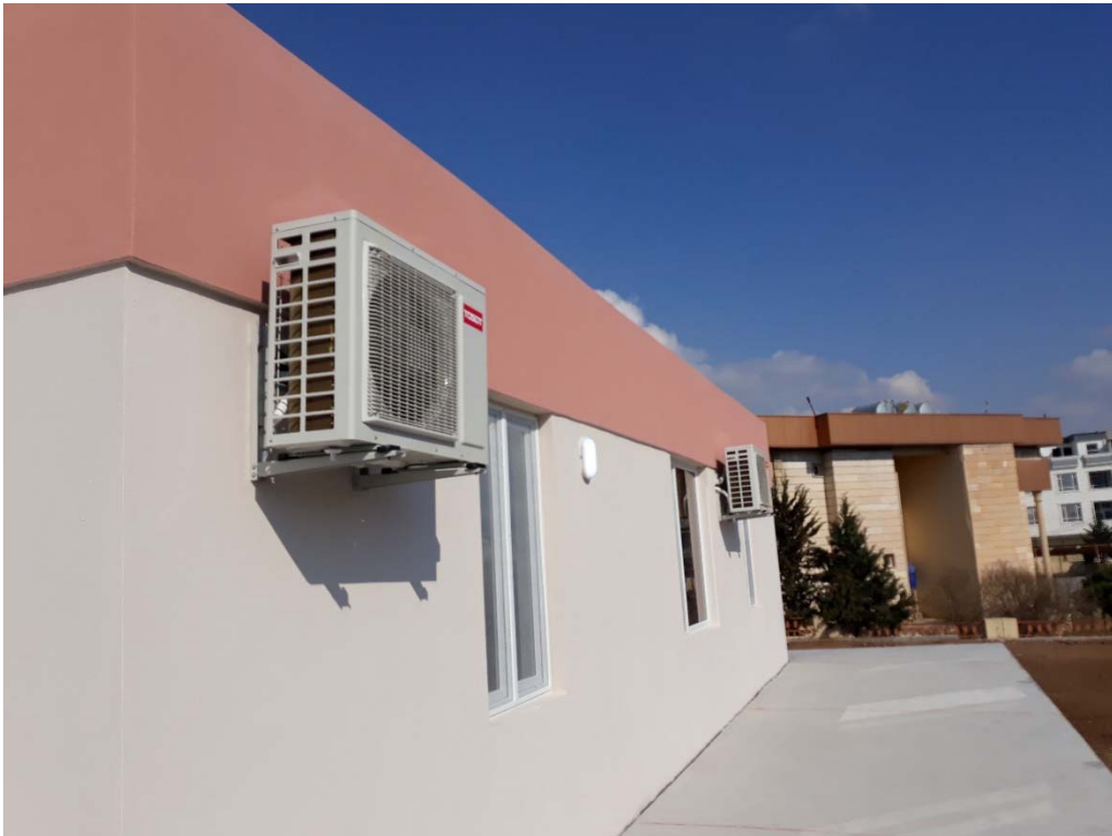
Main building - North side view
