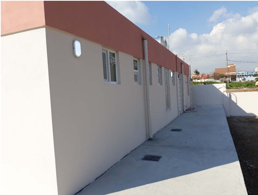
Main building-Backside view
