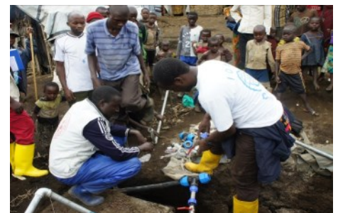
REHABILITATION OF A WATER SUPPLY NETWORK, NORTH-KIVU © IOM MAY 2017 (C.FRISONE)
