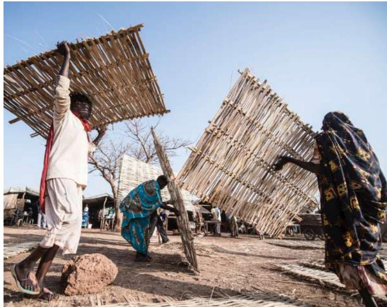
Construction of bamboo thatch walls for upgrading shelters through CBI, Wau PoC site, South Sudan, © R. Tupaz, IOM 2018
