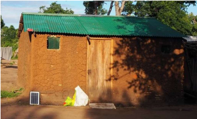
Figure 5: House with flat metal roof with mud and stick walls © IOM 2022
