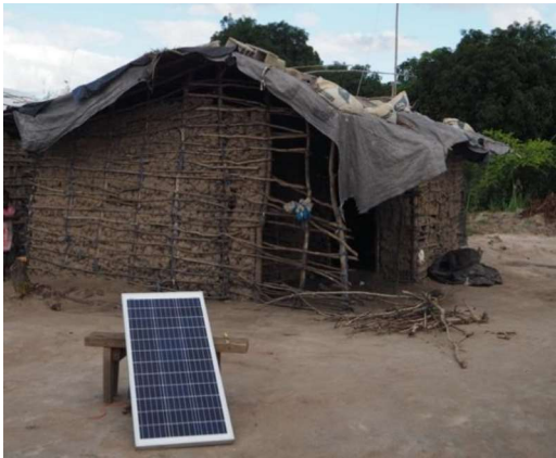
Figure 4: House with tarpaulin roofing with mud and stick walls © IOM 2022
