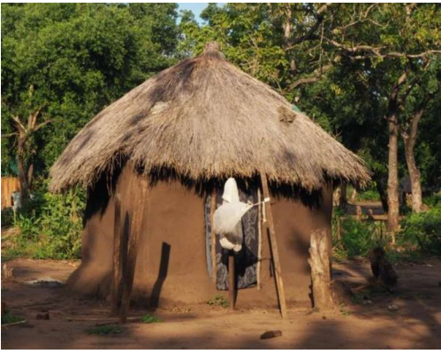
Figure 6: House with grass roof with mud and stick wall © IOM 2022
