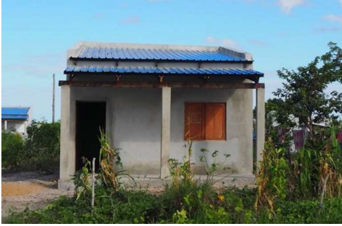
Figure 3: House with flat metal roofing with brick/concrete walls © IOM 2022
