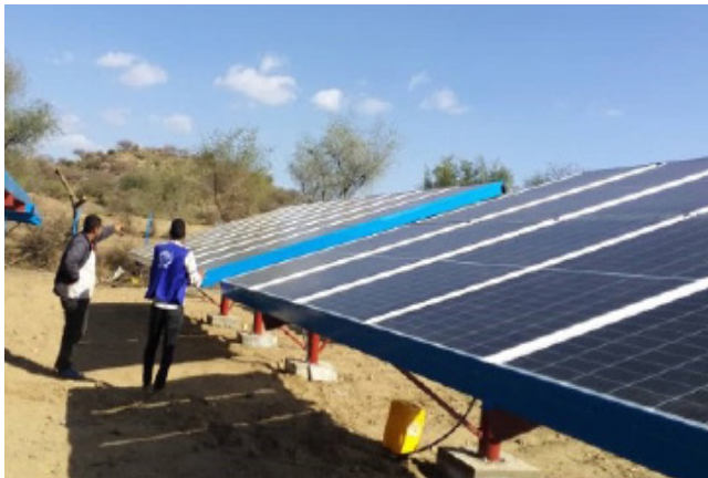
Al Al Mashawelah water site in Taiz Governorate using solar groundwater pumping ©IOM Yemen, 2021
