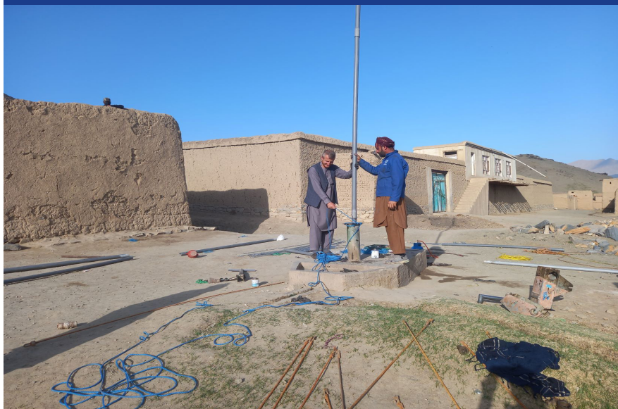
IOM's ongoing rehabilitation of boreholes in Afghanistan, 2021 © IOM Afghanistan.
