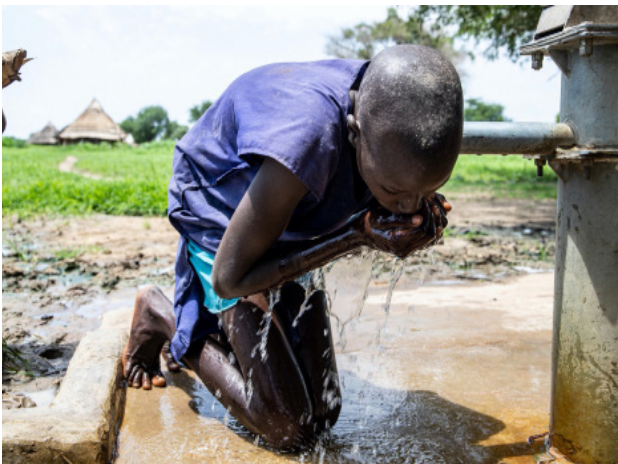
Nyalok Loongar drinking from IOM installed borehole in Thiet payam, Sudan @IOM Sudan, 2021
