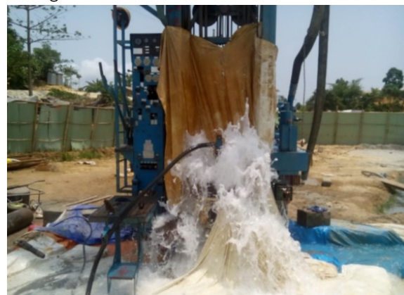
Figure 2: Airlifting in IOM Borehole Camp 12 - Kutupalong Mega-Camp, Cox's Bazar, Bangladesh
