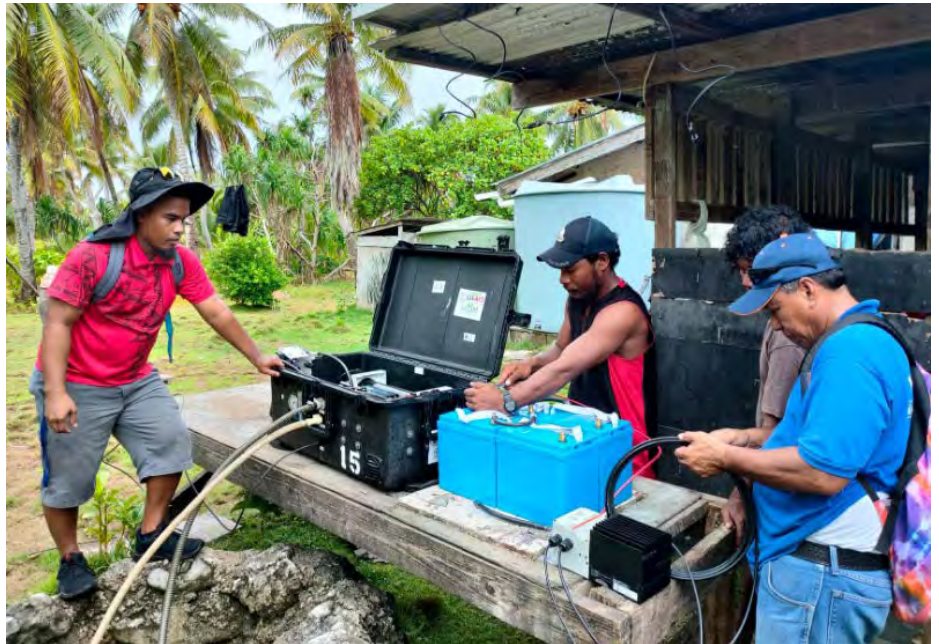
Technicians in RMI conduct maintenance checks on RO Units to prepare for upcoming drought seasons. Photo: IOM 2022
