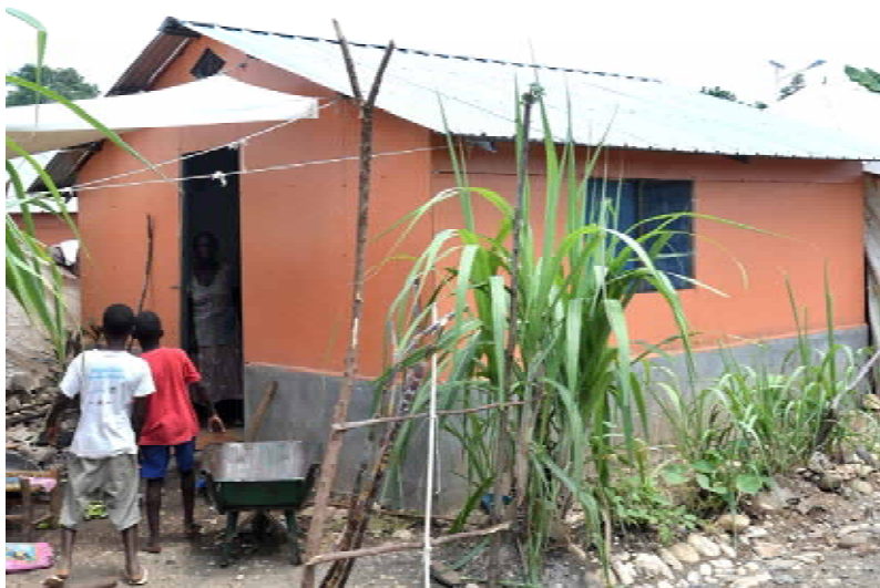
Above: Camp Mayard, Jacmel. IOM-built semi-permanent housing.
