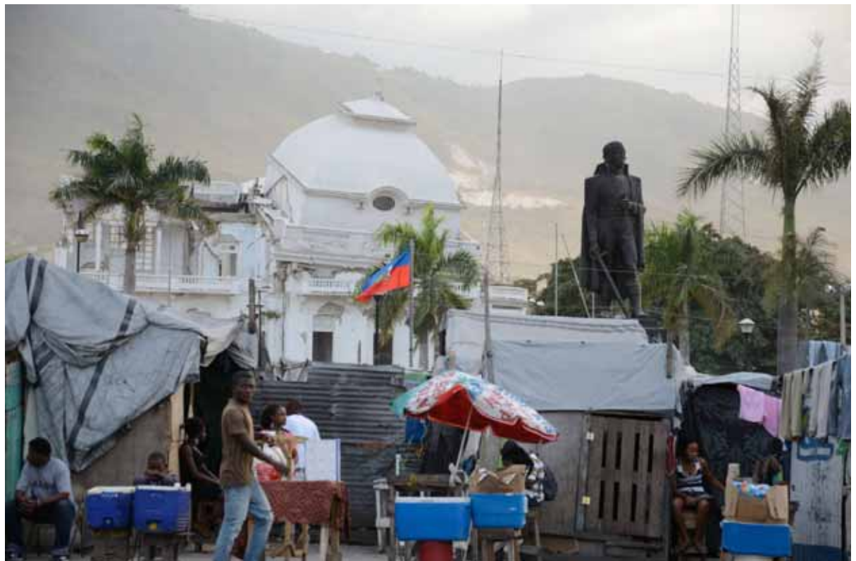
Right: Champs de Mars. The National Palace, damaged by the 2010 earthquake, faces a public square hosting displaced persons.
