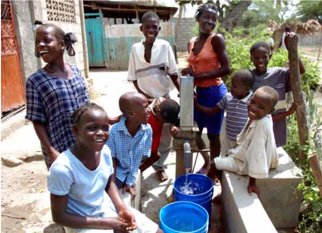
Left: Petit Goave. Hand pump installed by IOM.
