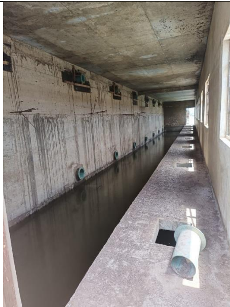
Photo 6: Flooded area at the filter gallery
