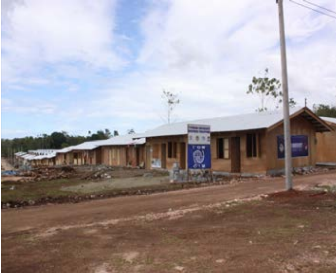
Bunkhouse Transitional Shelters
