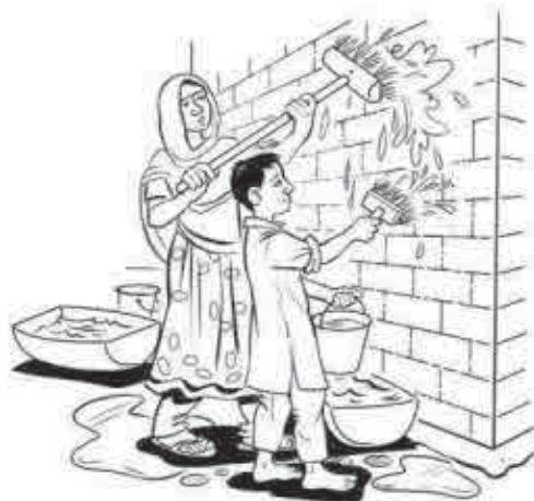
Fig 95- Wet the walls before applying render
