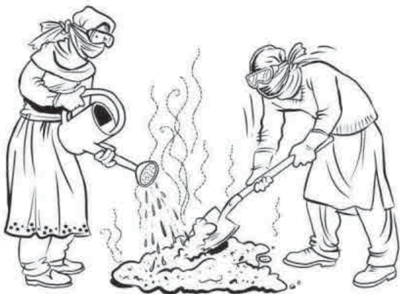
Fig 57: Hot Mixing - add minimum water
