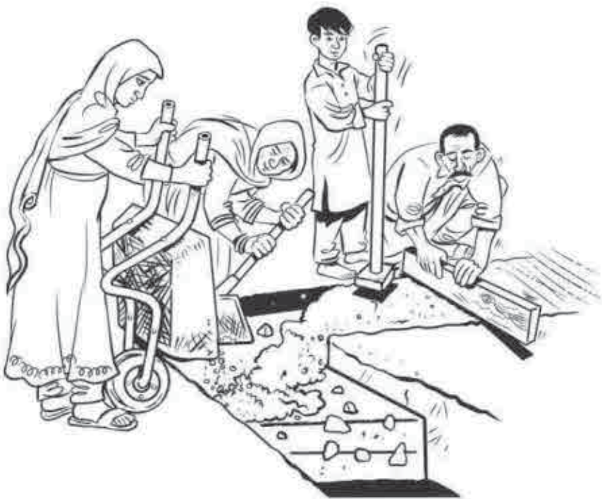
Fig 69: Good compaction is essential for foundations
