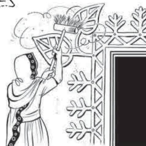
Fig 106: Brush down the walls to remove dust and debris, prior to wetting the walls and applying lime wash
