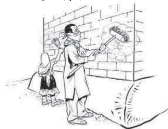
Fig 93: Brush walls to remove dust and debris
