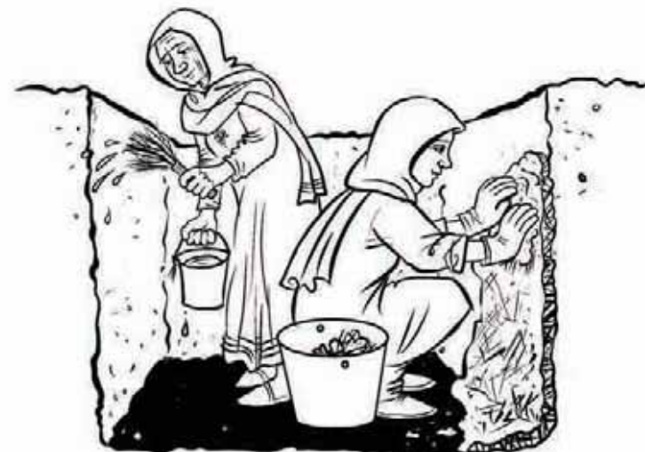
Fig 31: Lime Pit Preparation - Plastering the sides of the pit
