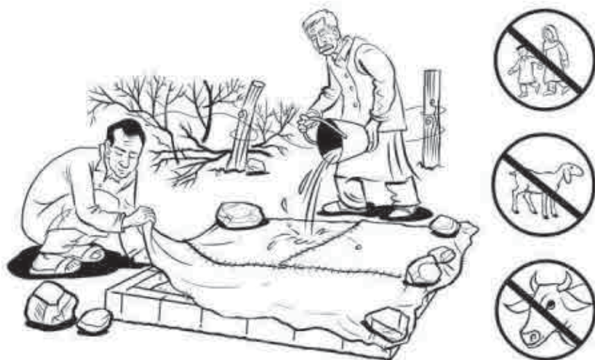
Fig 34: Keep the lime putty clean by keeping the putty settlement tank covered
