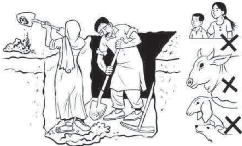
Fig 26 - Lime Pit Preparation - For safety keep children and animals away from the lime slaking and settlement pits
