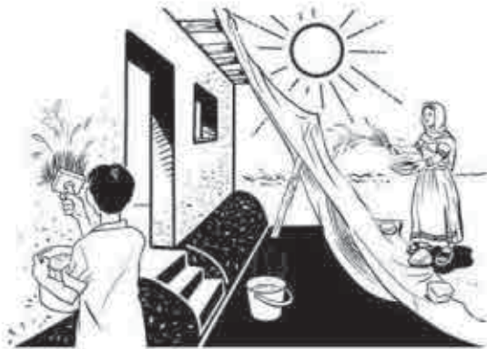
Fig 107: Wet the walls thoroughly half an hour so before applying lime wash: then again 5 minutes beforehand and leave to soak in, to ensure the porous background renders or plasters will not dry out the thin lime wash coats too quickly
