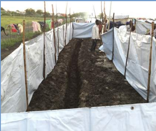
IOM-dug emergency trench latrine at Malakal PoC
